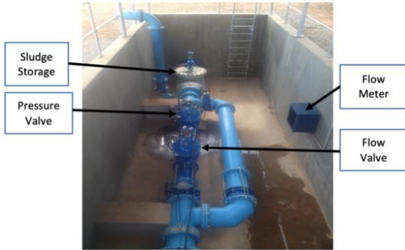
Figure 14 – Installed PRV
